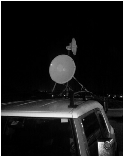
Figure 6 A roof mounted Mid Mile node
